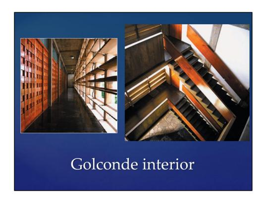
The doors and furniture are all made from Burma teak; the floors of black Kadappa stone; the white walls are made from crushed seashells, lime, egg whites and curd-known as Chettinad plaster, which is highly reflective.
